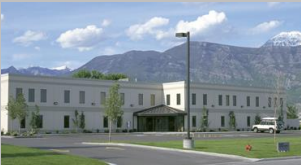
American Fork UT, USA Temperature
