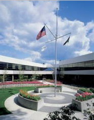
Everett WA, USA Electrical
