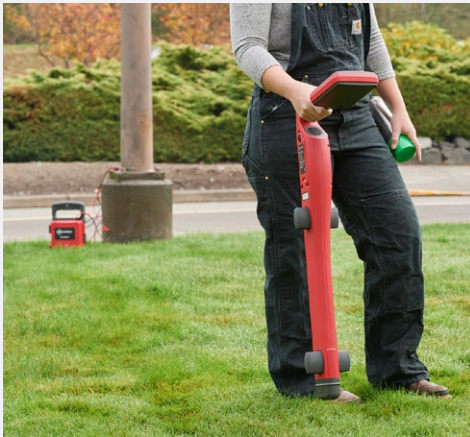
Trace an individual utility by connecting the transmitter directly with the test leads
